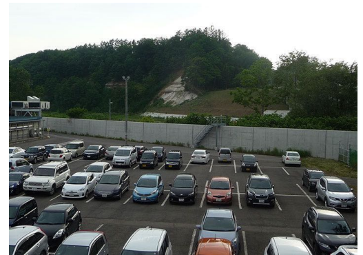
Nihon Kanzume water barrier
