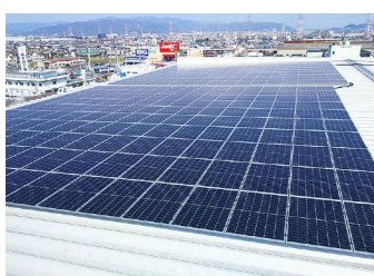
Meiji Oils and Fats (April 2020 Operation)
