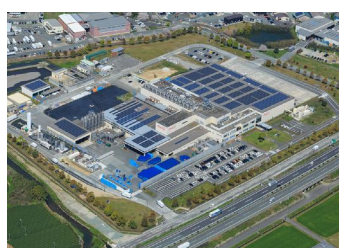
Kyushu Plant (April 2020 operation)
