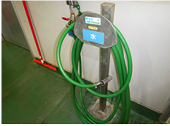
Meiji Co., Ltd., Asahikawa Plant, hose with water-saving nozzle
