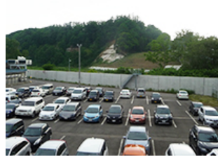
Nihon Kanzume, Co., Ltd., water barrier
