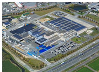
Solar power generation equipment, which started operation in April 2020 at Meiji's Kyusyu Plant
