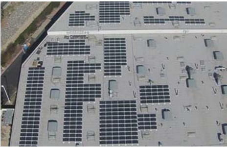
Santa Ana Plant
